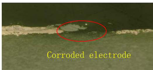
Figure 1 Left top terminal is corroded
